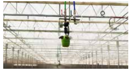
▲AKIMist® "E" Dry Fog humidifier with 4 nozzles attached
